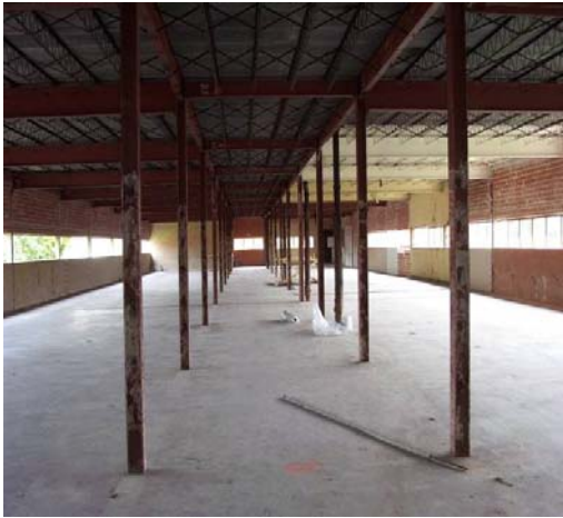
The Geology building interior before new construction.
